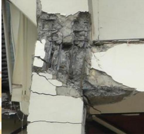
**Gambar 1. 2** Kerusakan Sambungan Balok Kolom Eksterior (<http://www.wm-site.com/civil-eng/short-course-haki-komda-bali-2010>)
