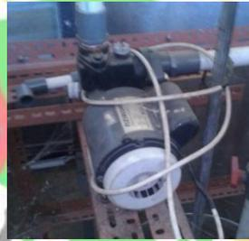
Gambar 3.7 Pompa air.
