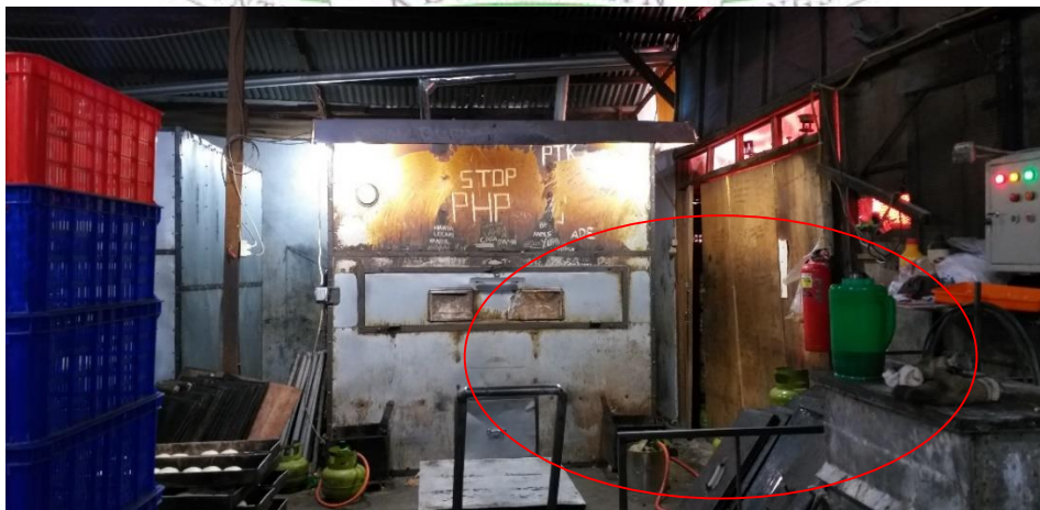
(d) Storage of gas cylinder is near the oven
