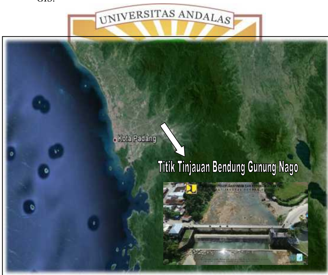
Gambar 1.2 Lokasi Penelitian Hulu DAS Batang Kuranji(sumber: google earth).
