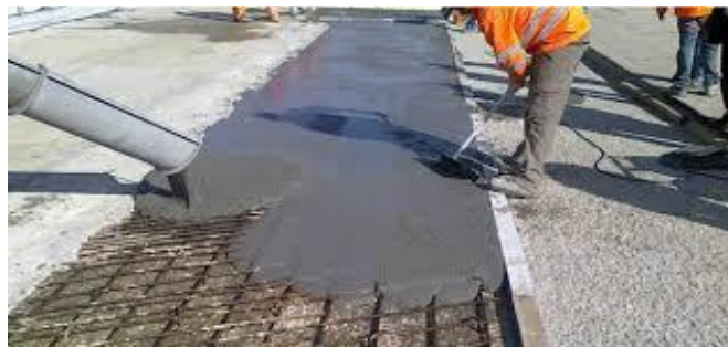
Gambar 1. 1 Beton Self-Compacting Concrete (SCC)
