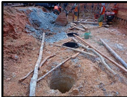
Gambar 4.6 Pemasangan Casing Bore Pile
