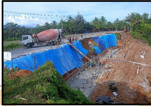
Gambar 4.8 Pengecoran Bore Pile
