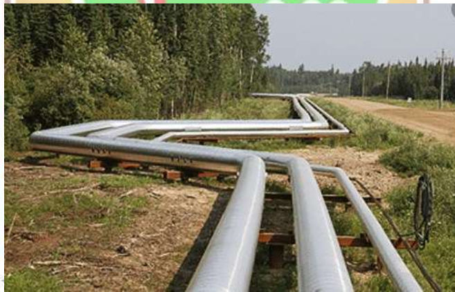
Figure 2. 1 Expansion loop
