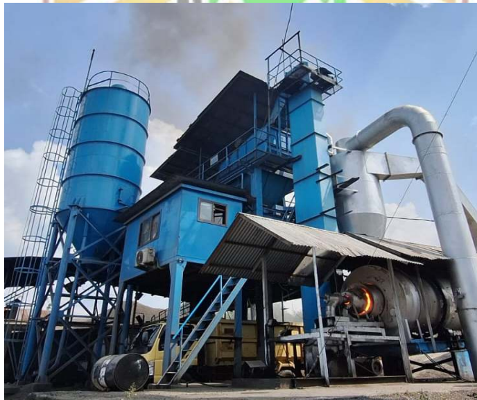
Gambar 2.14 Asphalt Mixing Plant
