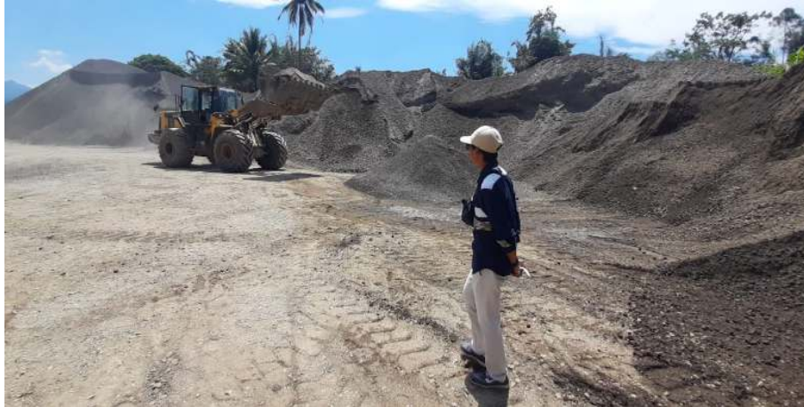
Gambar 4.7 Pencampuran/blending material aggregate kelas A
