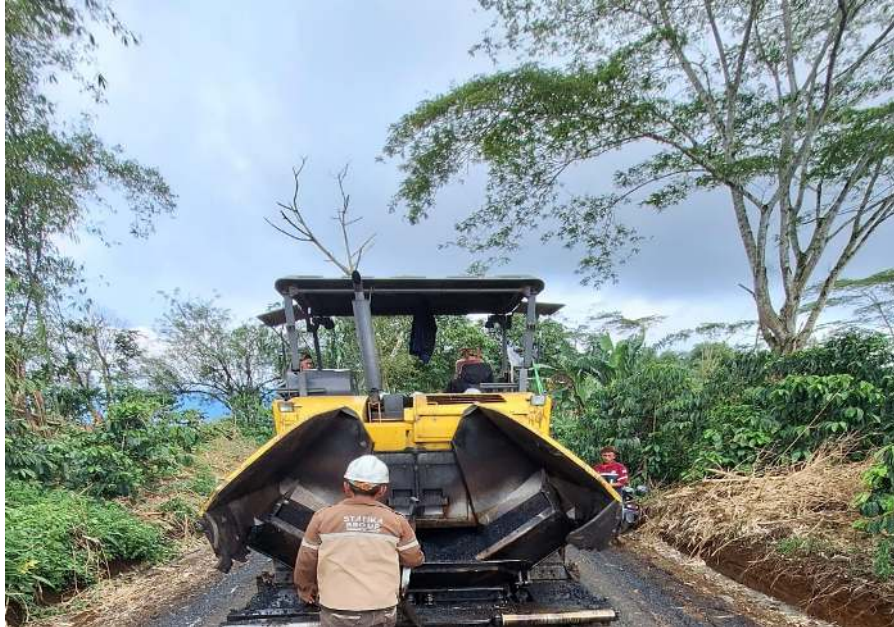
Gambar 4.12 Hopper asphalt finisher
