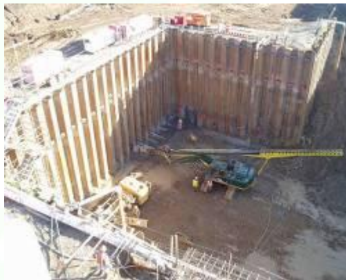
Sheet pile wall
