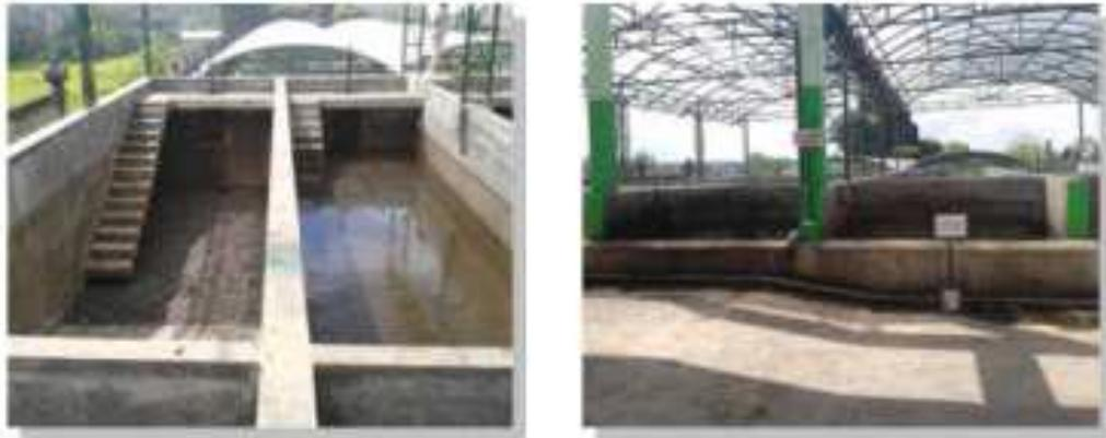
**Gambar 2. 7 Unit Solid Separation Chamber**
