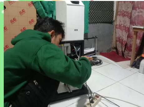
Pemasangan housing box
