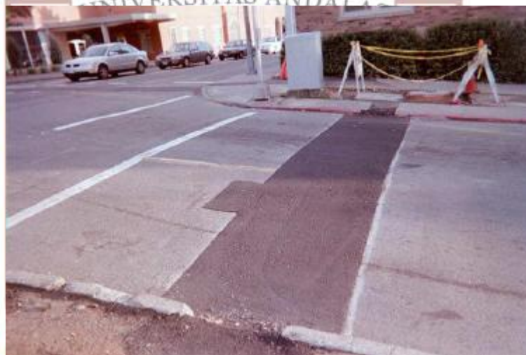
Gambar 1.17 Tambalan dan Tambalan Galian Utilitas ( Patching and Utility Cut Patching )
