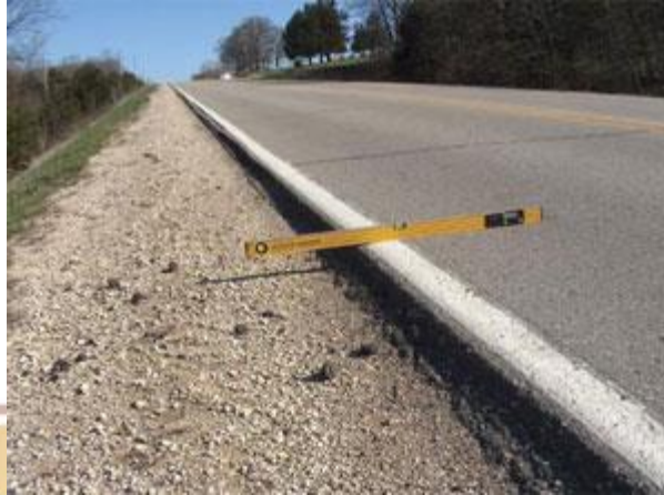
Gambar 1.12 Jalur/Bahu Turun (Lane/Shoulder Drop-off)
