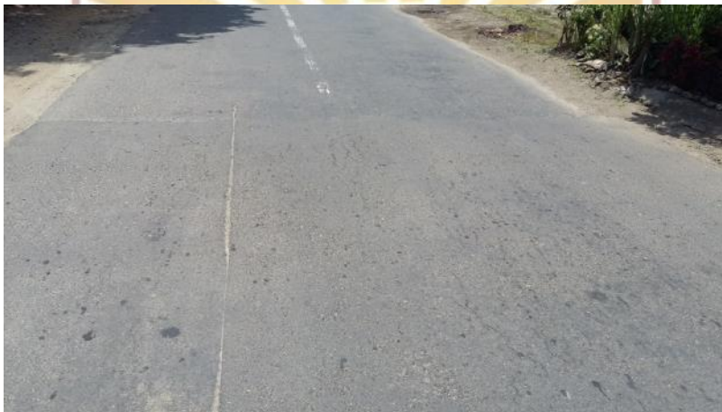
Gambar 3.2 Patching & Util Cut Paeth (Tambalan) (11L)
