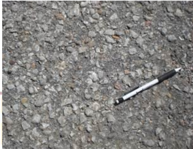
Gambar 1.13 Pelapukan dan Butiran Lepas (Weathering and Raveling)
