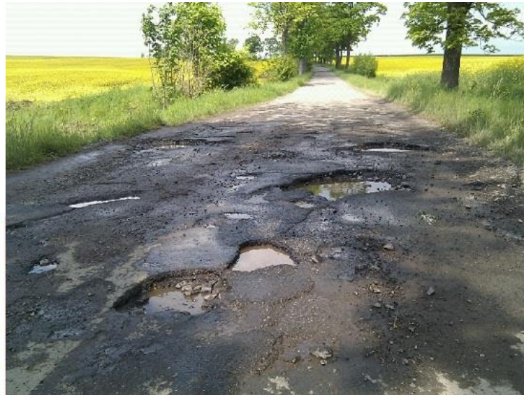
Gambar 1.16 Lubang (Potholes)
