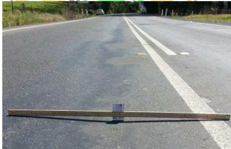
Gambar 1.2 Alur (Rutting)
