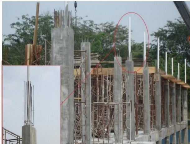
Figure 1.1 Pipelines on Hollow Reinforced Concrete Column
