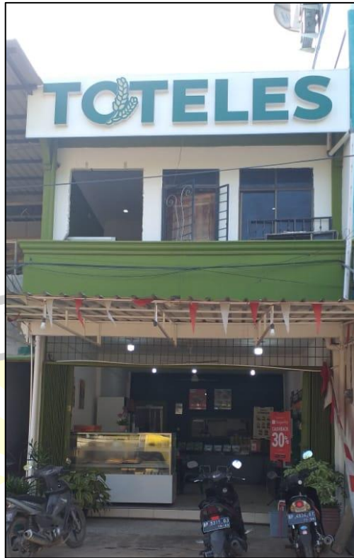
Figure 1.2 Building of Toteles Food and Bake House
